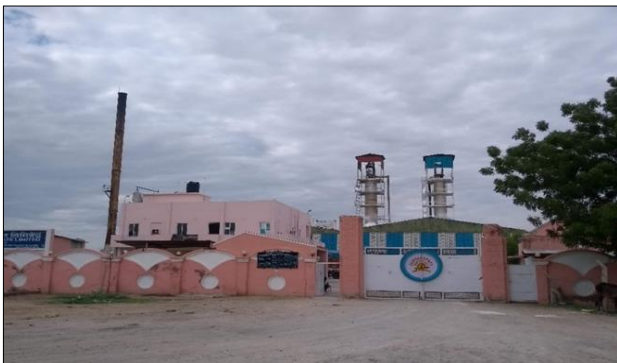
Fig 7: Chemical factory present in study area
