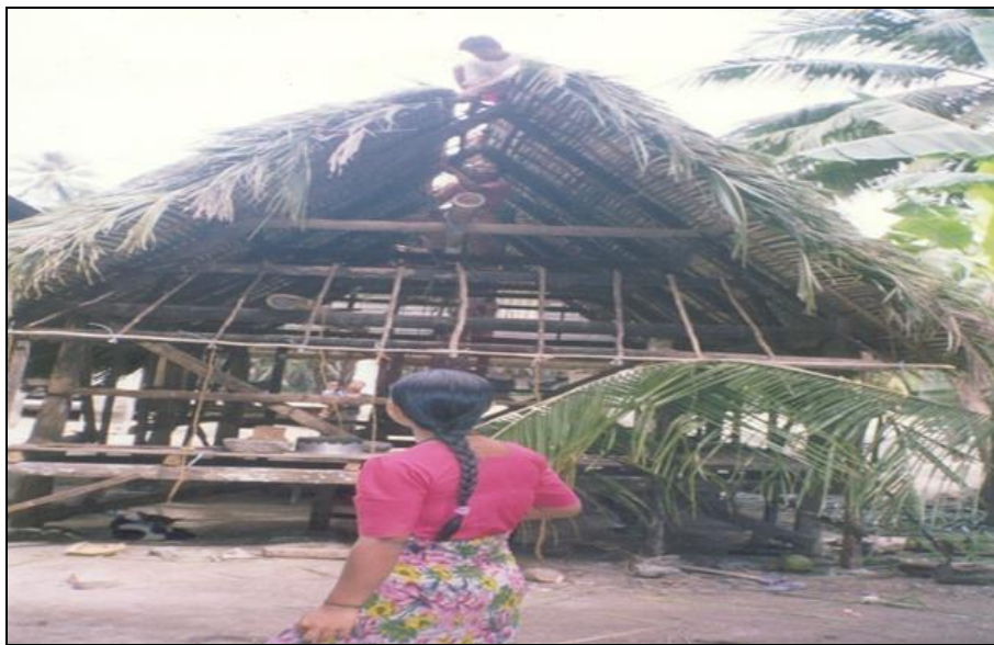
Plate 2: Nicobari couple thatching their hut using coconut leaves
